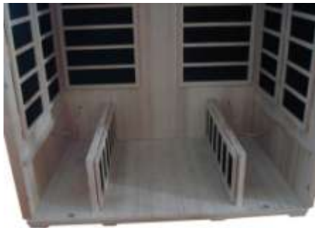
Figure B-4: Installing the bench stand panels
