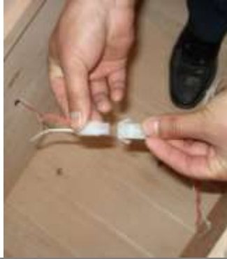
Figure C-5: Connecting the heater's plug
