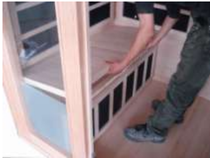
Figure B-7: Installing the benches
